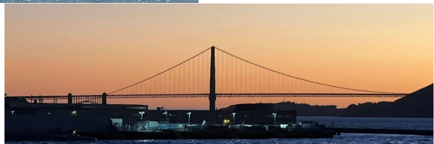
Golden Gate Bridge, San Francisco
